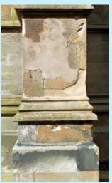
much repaired, often badly. Sandstone is porous and will therefore absorb rain water. This evaporates in dry weather, but over time the continual repetition of this process weakens the rock and parts of the surface may break off. Here, on the east side, cement mortar has been used to repair the surface of the stones. This is less porous than the stone and also stronger. Consequently it has trapped moisture
